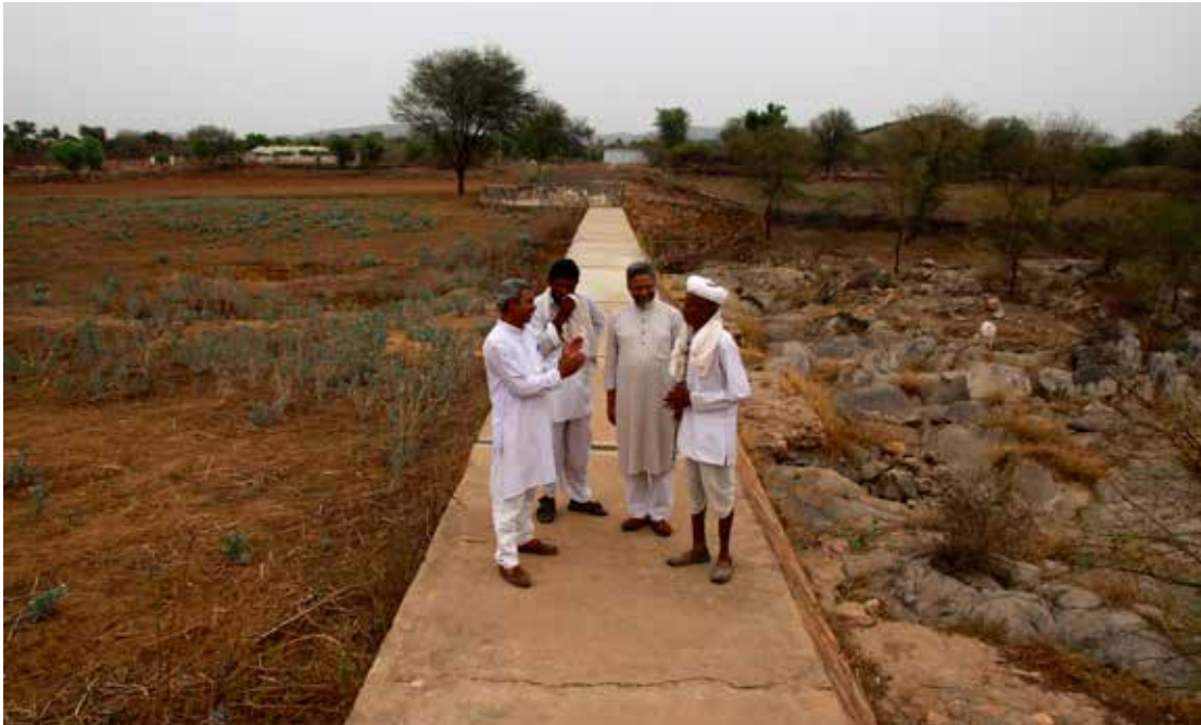
Inspection of a RWHS .
